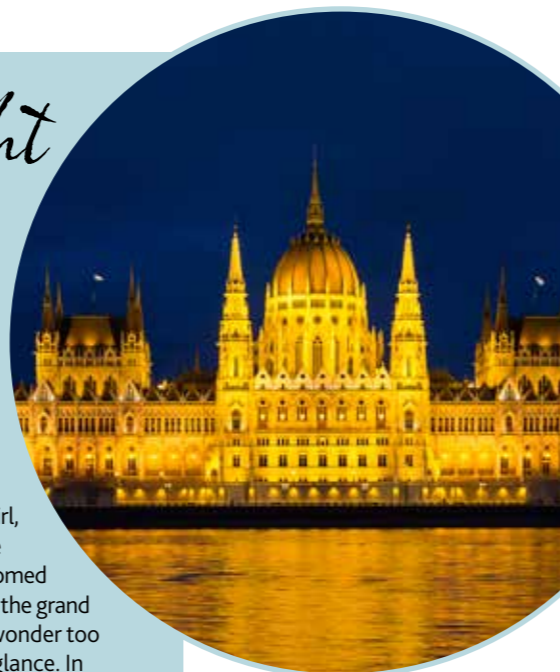
ABOVE The Gothic Revival-style Hungarian Parliament on the bank of the Danube – it is the country's largest building. BELOW Parliament's ornamental Grand Staircase, complete with frescoes and royal statues
